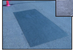
Firm-Grade on Parking lot
